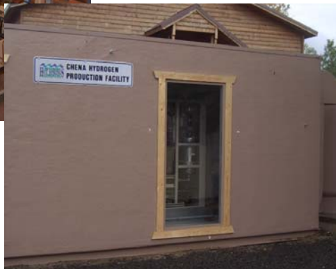
Hydrogen Production Facility at Chena
